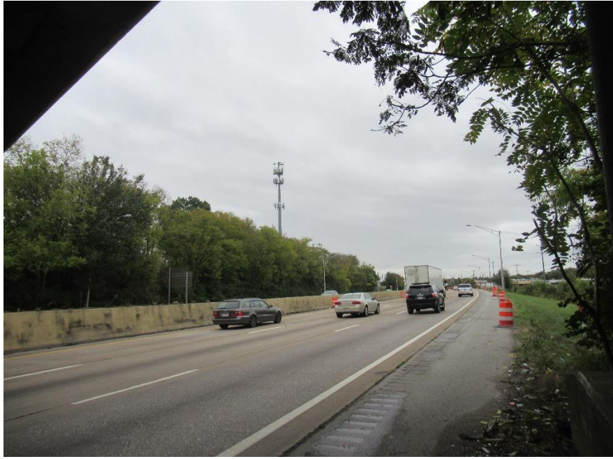
LOOKING AHEAD ON ROUTE FROM UNDERPASS - EASTBOUND
