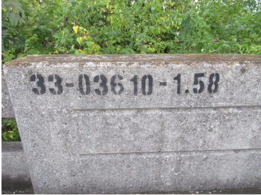
BRIDGE NO. - BRIDGE RAIL - #1 RIGHT SIDE
