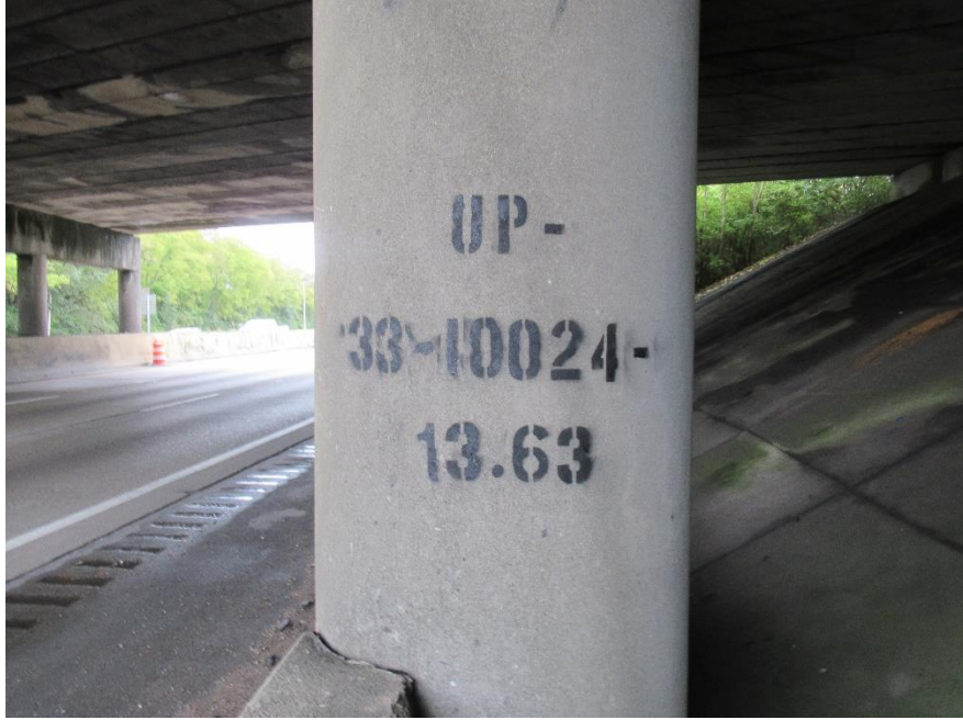
UNDERPASS NO. - BENT #1 - COLUMN "B"
