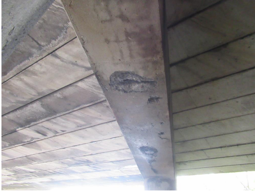
BOTTOM OF CAP - BENT #1 - BETWEEN COLUMNS "D" AND "E"
