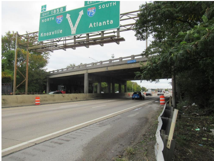
LEFT SIDE VIEW OF BRIDGE
