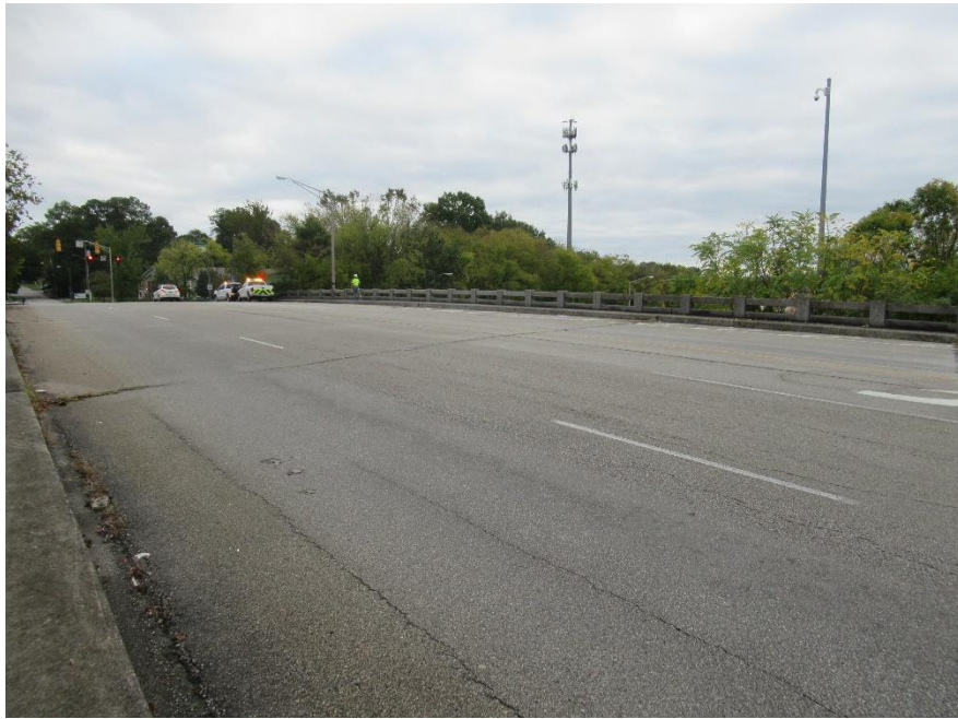
VIEW ACROSS TOP OF DECK
