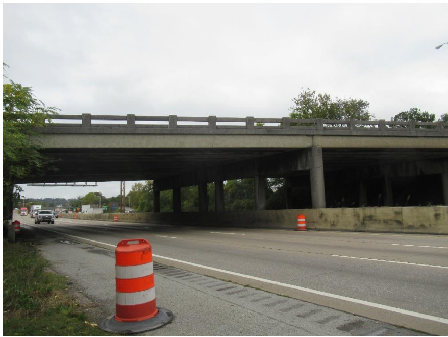
RIGHT SIDE VIEW OF BRIDGE
