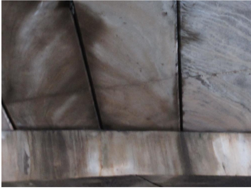
BEARING "L" - ABUTMENT #1
